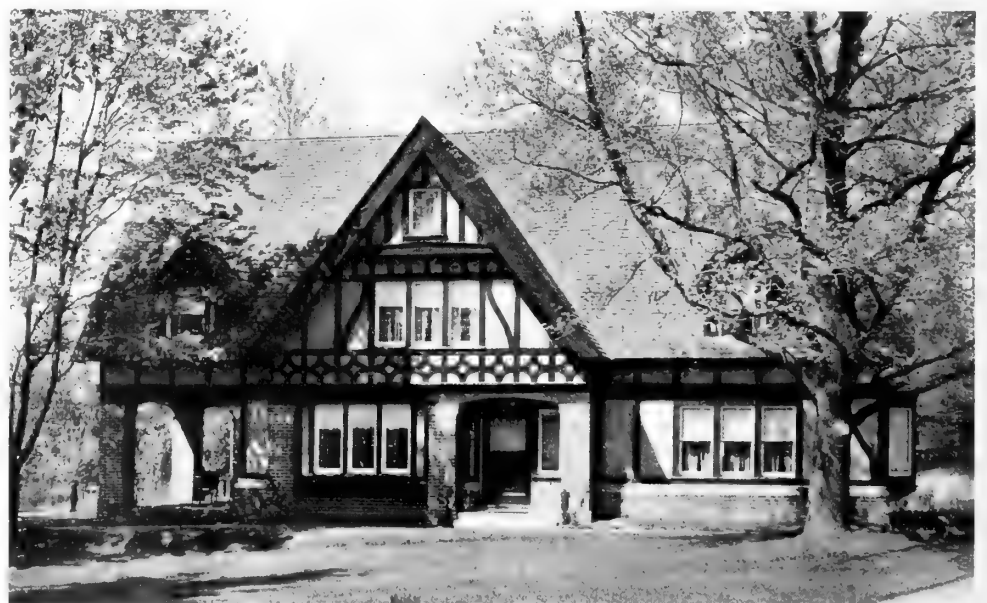
9—Harvard Brick, Beams and Stucco are the Materials Used for the Exterior of the House
